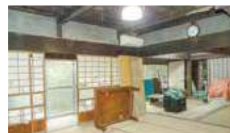
“紬”-tsumugi-改修前の室内
